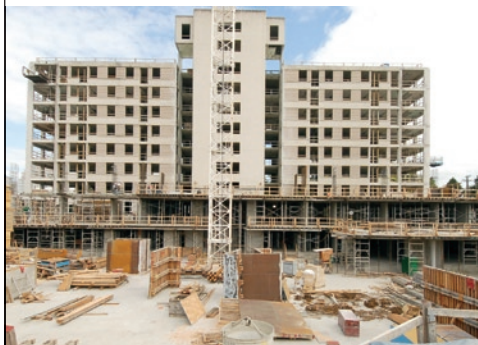
Tapestry, July 2006: In background, 10-storey building being retained and renovated. In foreground, construction of new section of 10-storey building
