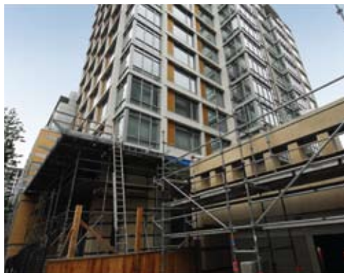
The Patina highrise in downtown Vancouver is progressing well
