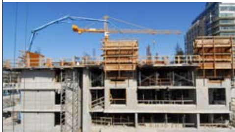
Concrete work is nearing completion at Tapestry at Wesbrook Village UBC
