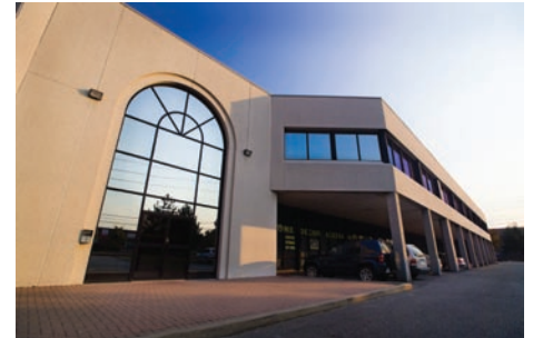
6625 - 6705 Tomken Road, Mississauga, ON
