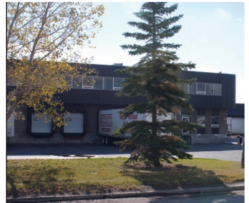
4747 54th Avenue, Calgary, AB – 100 per cent leased industrial building
