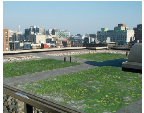
Eighth floor extensive green roof at Jazz, Toronto, ON
